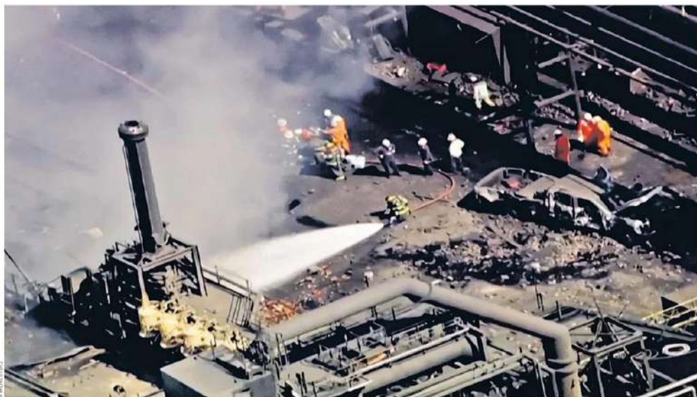
DEVASTATION: Firefighters at the site of a blast Monday at Clairton Coke Works, southeast of Pittsburgh, in an image taken from video. Two people were confirmed dead and 10 others were injured. For video, scan the code with the article on A3.
